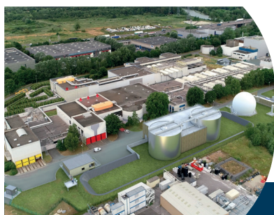
Wastewater treatment plant Saint-Thibault-des-Vignes (77) - 350,000 E.H. Energy recovery from sludge and biogas injection
