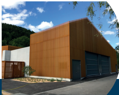
Delémont wastewater treatment plant (Switzerland) - 39,000 p.e. Micropollutant treatment (CarboPlus® wastewater)
