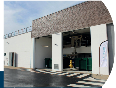
Coulommiers drinking water plant (77) Fluorine and strontium treatment and strontium
