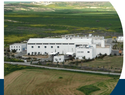
Vathia-Gonia wastewater treatment plant Vathia-Gonia (Cyprus) - 200,000 E.H. Reuse of treated wastewater (Aqua-RM® membrane treatment)
