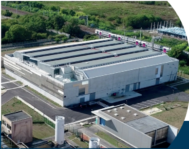
Orly 2 drinking water production plant (94) - 150,000 m 3 /d Treatment of organic matter (Delreb®), and micropollutants (CarboPlus® drinking water)
