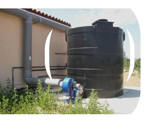
As a true alternative to conventional odor control methods such as physico-chemical scrubbing or activated carbon, LANODOR® can serve as a complementary solution for pretreating effluents with high concentrations of hydrogen sulfide, reducing chemical reagent consumption and operating costs.
