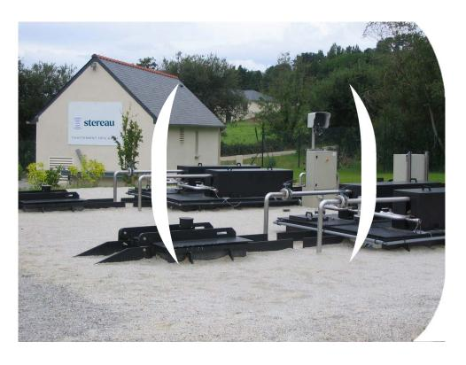
Based on the **AQUA-RM®** process, which combines biological treatment by activated sludge and filtration by submerged flat sheet membranes, **COMPACT-RM®** is a complete, modular, upgradeable and standardized plant.
